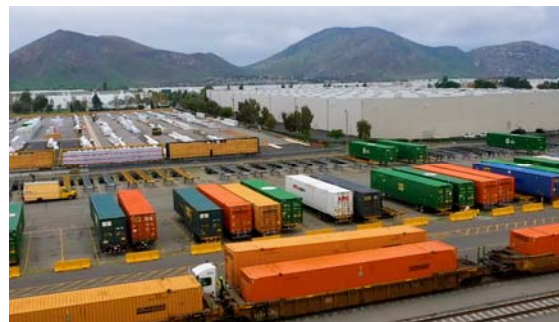
Inland Empire Intermodal Terminal Colton, California
