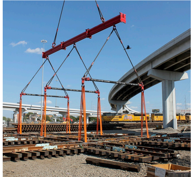
A crane prepares to move the new diamond into place Aug. 9.
