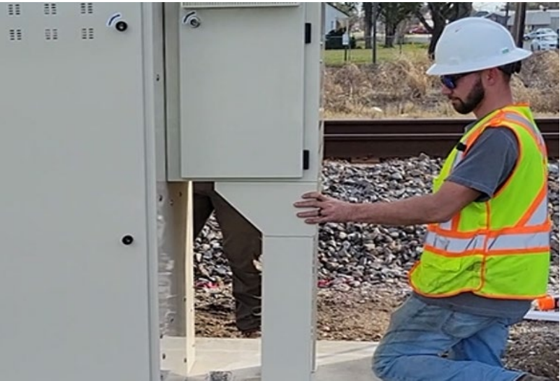
A hydrogen supplier installs a new hydrogen-powered fuel cell at a Union Pacific crossing in Louisiana.
