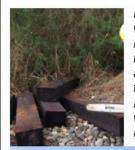
Field cuts are made to wood timbers out of necessity, yet they breach the treated layer of wood and open up a pathway for fungi and insects. Recovering the cut area with preservative will seal it and prevent decay.
