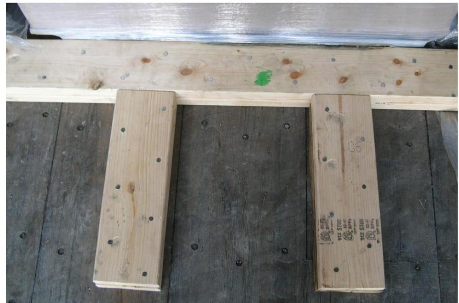
**Floor blocking should be constructed with double 2x4 or 2x6 lumber with backup cleats, at least 18 inches long. Floor blocking needs to be as long as the pallet or unit it is supporting. Nails should be staggered and spaced approximately 4 to 5 inches apart. 16d nails (or larger) are required.**
