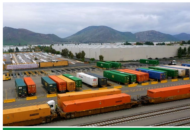
Inland Empire Intermodal Terminal (IEIT), Colton, California.
