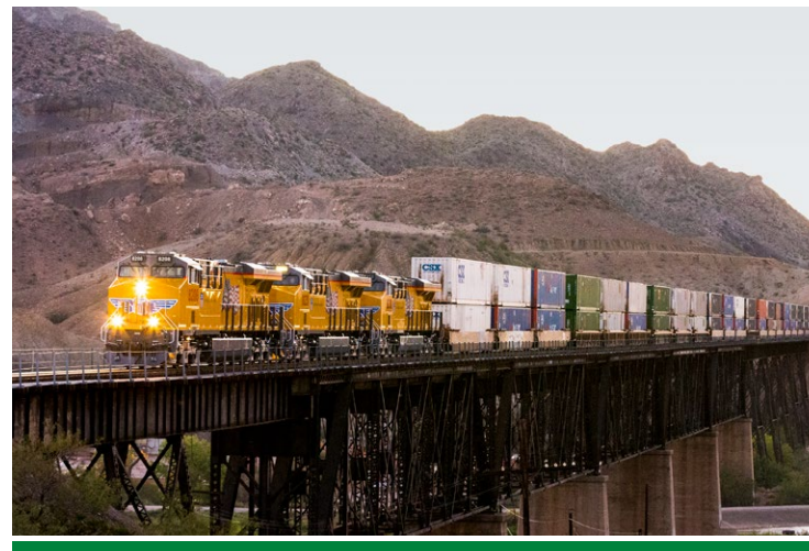
Intermodal train on the Golden State route near El Paso, Texas.
