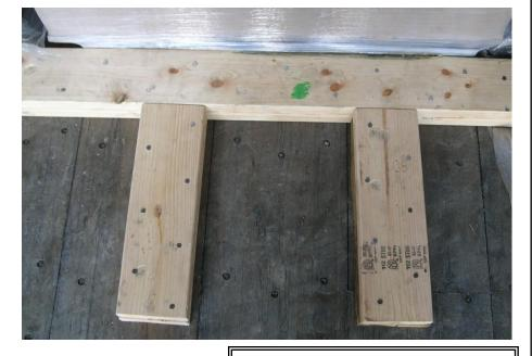
Floor blocking should be constructed with double 2x4 lumber with backup cleats, at least 18 inches long. Floor blocking needs to be as long as the pallet or unit it is supporting. Nails should be staggered and spaced approximately 4 to 5 inches apart. 16d nails (or larger) are required.
