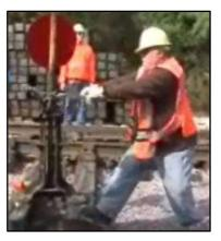
Employees are required to switch track junctions to redirect the direction of a train. This is done by pulling the track switch, or high stand switch. Applicants must demonstrate the ability to apply sufficient force to the switch by pulling in a horizontal direction on the testing device.
