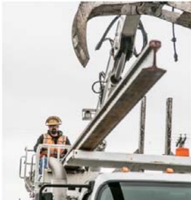
Automated Rail Unloading
