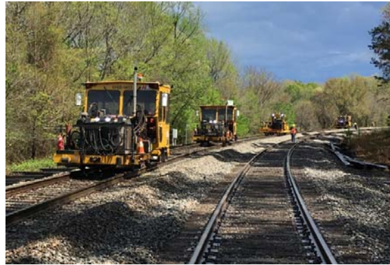
Wood Tie Renewal Operations
