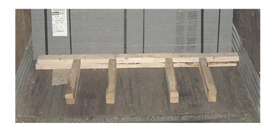
FLOOR BLOCKING SHOULD BE CONSTRUCTED OF DOUBLE LAMINATED 2x6 LUMBER WITH BACK UP CLEATS AT LEAST 18 INCHES LONG. NAILS SHOULD BE STAGGARD AND SPACED APROXIMATLY 4 TO 5 INCHES APART.
